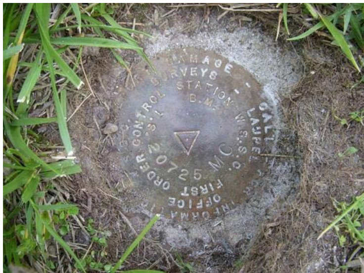
Figure 2.7: Finished product of a slightly weathered brass survey disk set in concrete monument.
